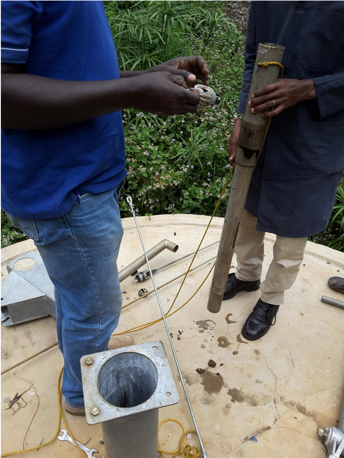
Rehabilitation works at Isinya Sampin spring. Spring had shallow constructed nearby. Working together with AMREF Technicians and with permission from German Agro Action, the shallow well was restored to working order.
