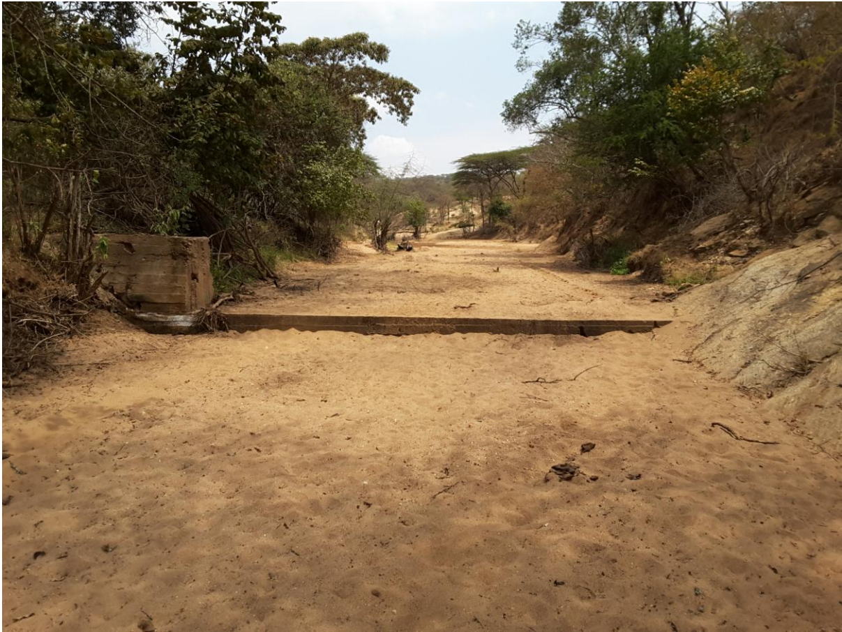
Matured newly repaired sand dam at Enkorika, Dalalekutuk Ward. This was one of the sand dams that were repaired after the El Nino rains.
